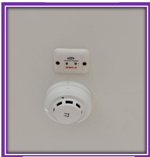
Smoke Detector and Temperature Sensor
